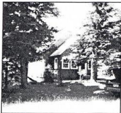
Rahko Home, now owned by Elma (Lampi) Olewinski on Misery Bay Road and Church Road.
