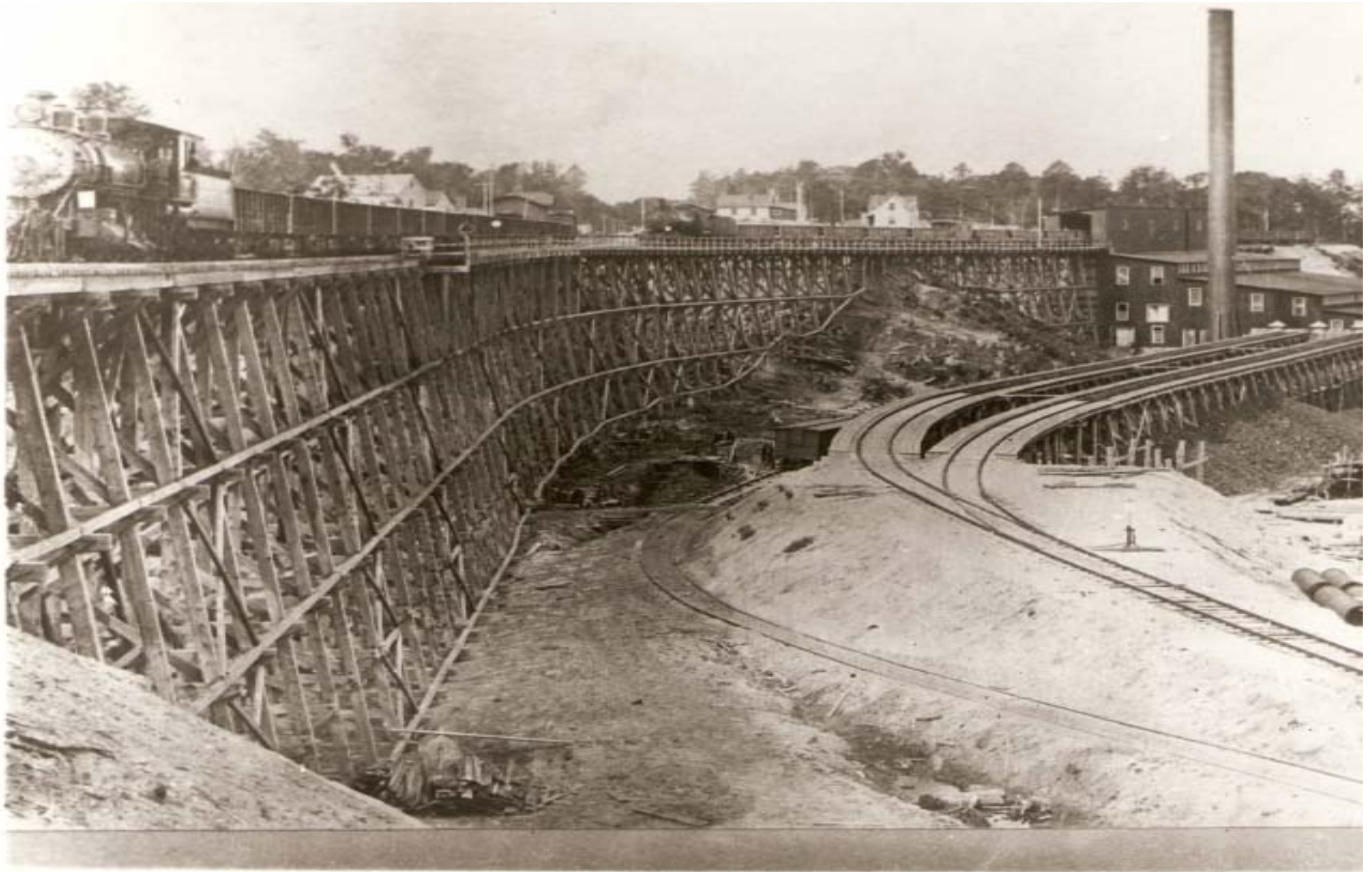
Trimountain Mill Wood Trestle Built in 1902; Rebuilt with steel in 1908; Mill Burned in March of 1916 Sincock Collection/B. Brinkman; Sharrar Collection
