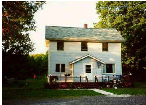
Copper Range Section House in Toivola, built in 1900
