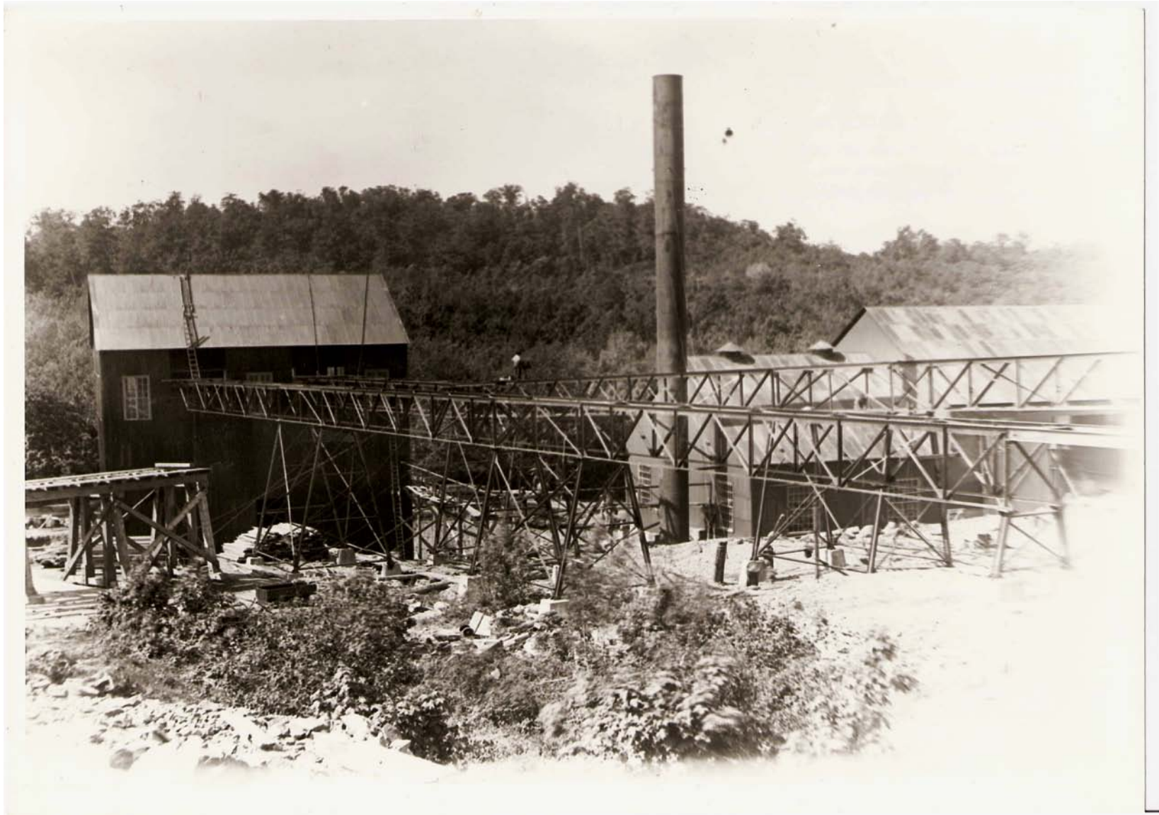
Barnes/Sincock Collection; J. Sharrar Collection Adventure Engine House & Hoist; 2/14/1902
