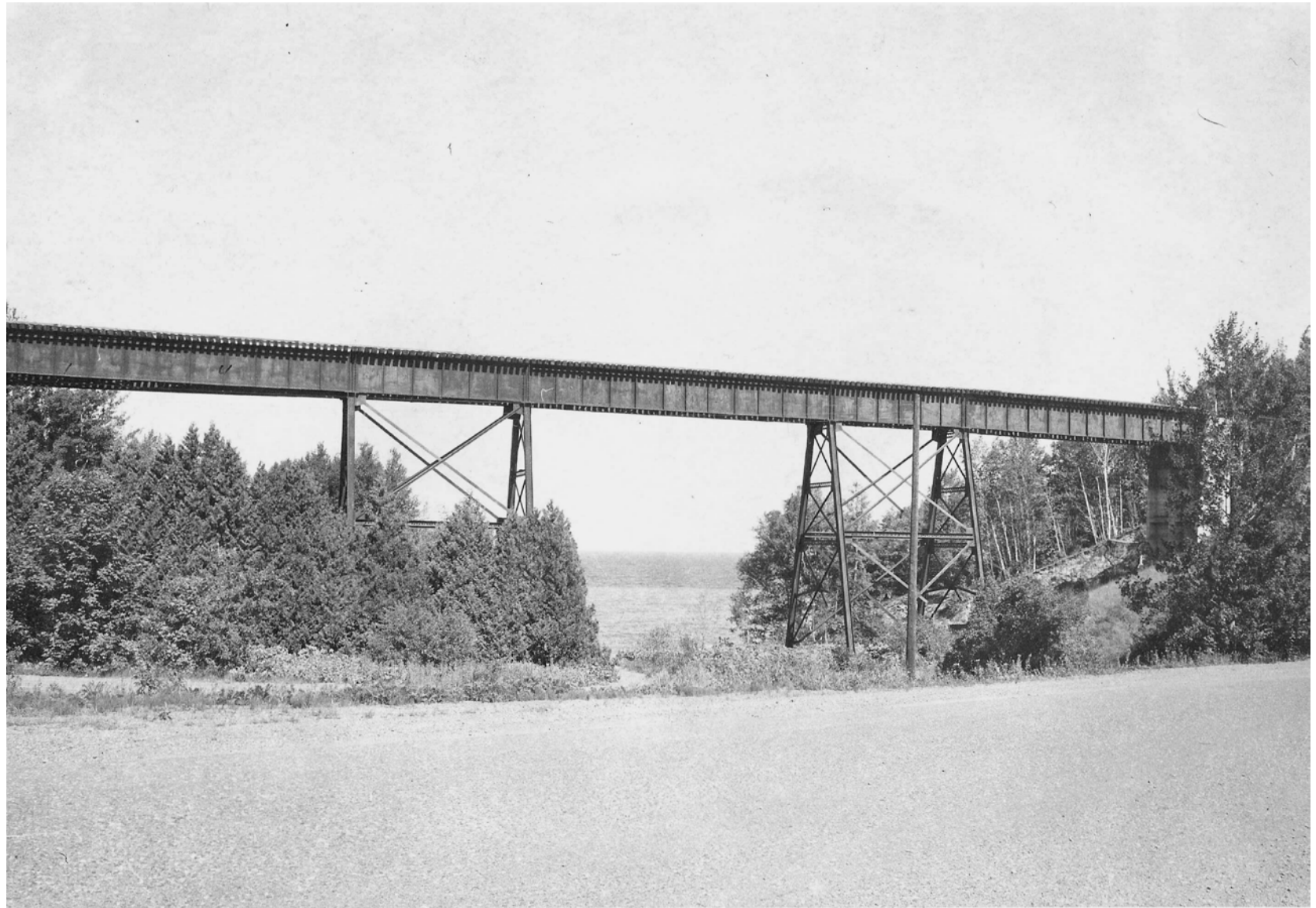
B. Brinkman Photo; J. Sharrar Collection 9/10/1971 Beacon Hill Trestle
