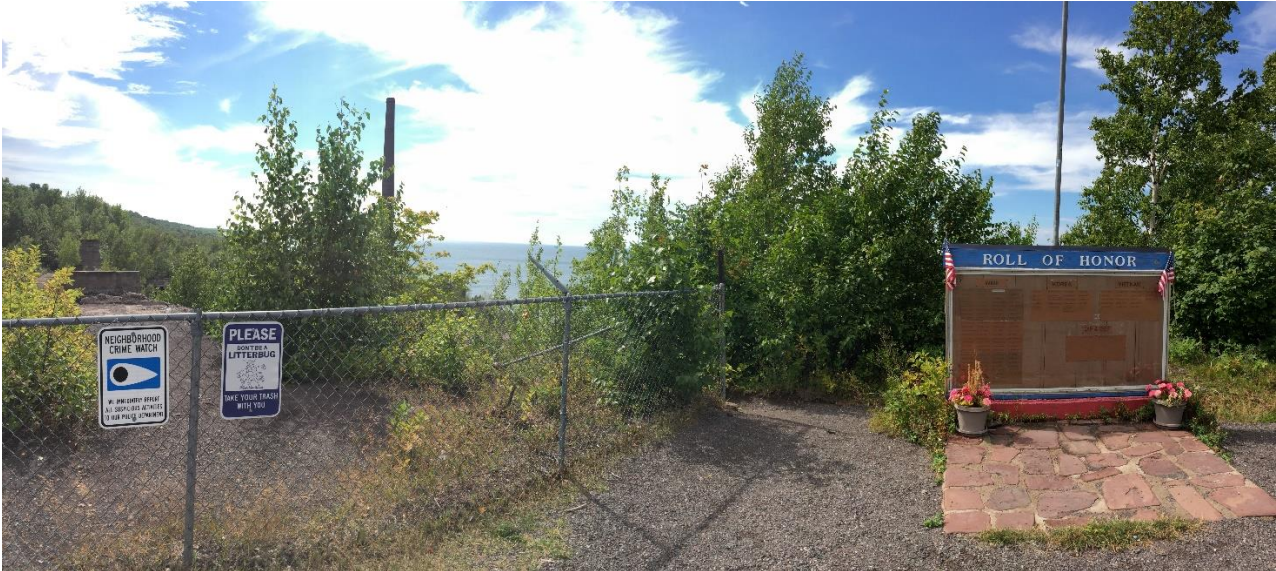
Figure 12. Freda Honor-Roll Memorial on the east end of the Park. Looking southwest toward ruins of the Champion Copper Stamp Mill (smokestack and Lake Superior in background).
