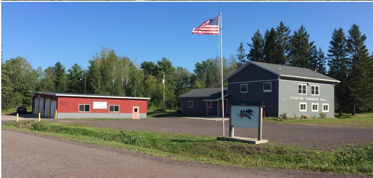
Figure 43. Stanton Township Hall and Firehall.
