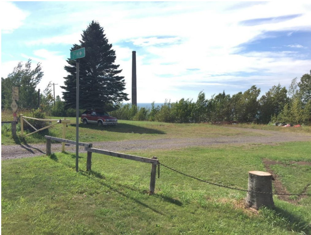
Figure 18. Former access route to shorelands of the Freda Honor-Roll Park and ruins of the Champion Copper Mill. This route is currently closed to the public.
